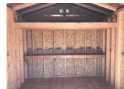
Loft Below Top of Wall
